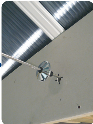
Fit the split rubber grommet and cover disc around the wire and feed into access hole
