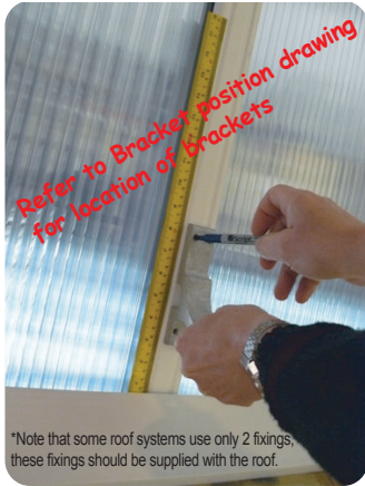
Use bracket as template to mark the position of the 4 holes*. Use a small pilot then open up with a 7mm drill bit
