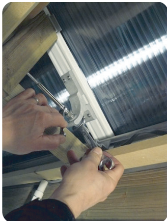
Use a 19mm spanner on the rear nut to tighten the assembly. Use an 10mm spanner on the flat to stop the wire from turning
