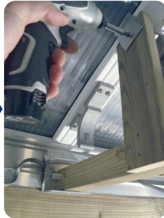
Construct the internal bulkhead system (Valance shown).
