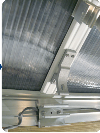
Secure using the M6 nuts and bolts provided. Ensure the nylon washer is underneath the nut to form a seal.
