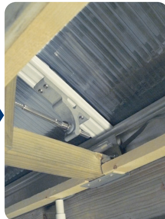
Adjust the wire tension by tightening equally at both brackets. Once taught, tighten the front nut against the bracket,
