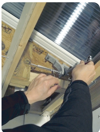
Use a 19mm spanner on the rear nut to tighten the assembly. Use an 10mm spanner on the flat to stop the wire from turning
