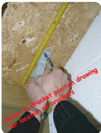
Use bracket as template to mark the position of the 4 holes. Use a 4.5mm drill to a depth of 75mm.
