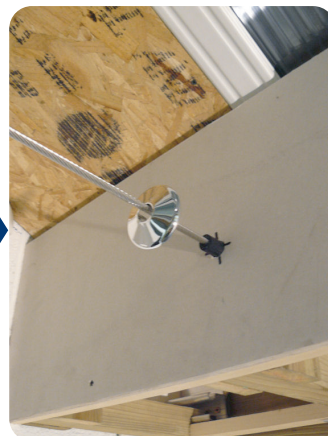
Fit the split rubber grommet around the wire and feed into access hole
