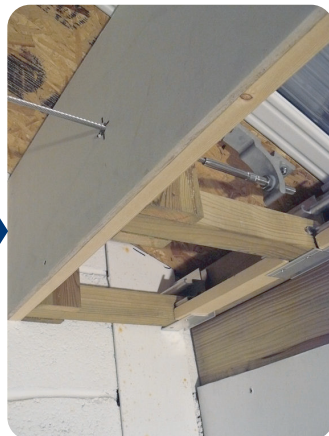
Adjust the wire tension by tightening equally at both brackets. Once taught, tighten the front nut against the bracket,
