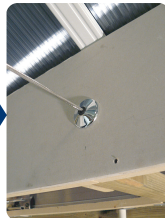
Fit the split chrome cover disc onto the rubber grommet to form a neat terminal on face of plaster
