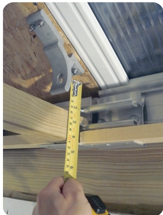
Measure from the bracket hole down to the underside of the bulkhead
