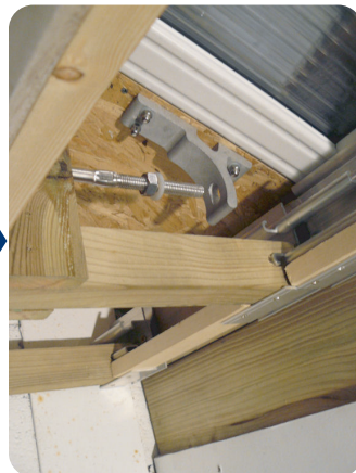
Remove the 2 nuts and washers from the ends of the Tiewire. Feed the wire through the access hole - reattach nut.
