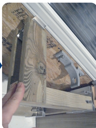
Construct the internal bulkhead system (Valance shown).
