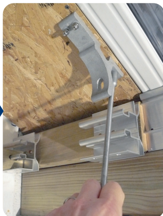
Secure using the 6x100mm dowel screws and washers provided. Drive screws through bracket via dome nuts.
