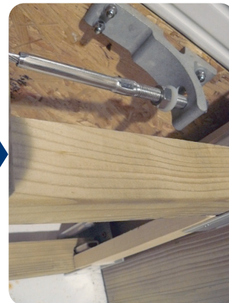
With 1 nut and washer in place, feed the wire through the slot in the bracket. Loosely attach rear washer and nut.
