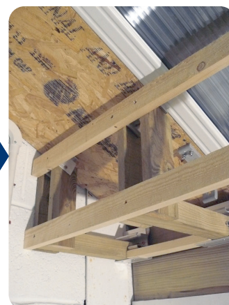
Complete the framework and ensure Tiewire can gain access to the bracket
