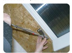
Bring the end of the wire with the tensioner across the roof to meet the **male** bracket. Offer the end of the tensioner (with the red spot) onto the threaded stud fixed to the male bracket. Rotate the tensioner onto the threaded stud of the male bracket, this will simultaneously draw in the terminal on the end of the wire. **DO NOT** allow the wire to rotate during this procedure.
