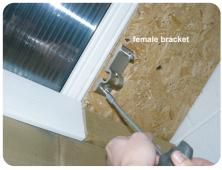
Secure the bracket loosely with the 4 dowel screws, hold the bracket in its final position and then tighten each screw until the bracket is tight and paralell to the timber. Do not over-tighten the screws or use an impact driver.
