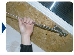
Final tension is achieved once the wire is straight and taut. Do not overtighten and allow the sides of the roof to become distorted. Tighten the locknuts against both ends of the tensioner body. Complete the installation by fixing the plasterboard. Mask of the brackets and protect the wire assembly during the wet plaster process.
