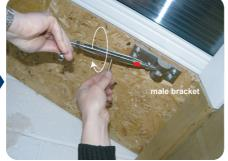
Keeping the wire terminal, tensioner and bracket stud in-line, continue to turn the tensioner until the slack is removed from the wire. **DO NOT** allow the wire to rotate during this procedure. Use a tool in the hole of the tensioner to apply the final turns. A 10mm spanner on the flats of the wire terminal will stop the wire from rotating.
