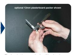
The bracket is secured using 4No. dowel screws. Optional nylon bushes are provided to pack the bracket off the surface of the timber and allow the bracket to sit flush with 12mm plasterboard.
