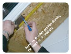
Refer to the bracket position drawing for the location of the brackets. Use bracket as template to mark the position of the 4 holes.
