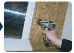
Use a 4.5mm dia. drill bit through the marks on the timber. Drill square to the surface of the timber to a depth of 75mm.
