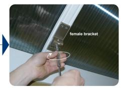
Identify that the wire has a short terminal at one end. Thread this terminal through the slot in the **female** bracket and into the bracket pin. Ensure the wire terminal is screwed fully into the depth of the threaded hole within the pin.
