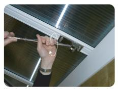
Keeping the wire terminal, tensioner and bracket stud in-line, continue to turn the tensioner until the slack is removed from the wire.
