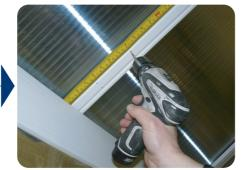
Use a small pilot drill through the marks on the rafter into the glazing channel. Open up the holes using a 7mm diameter drill bit. Attach both brackets to the opposing rafters using the fixings supplied
