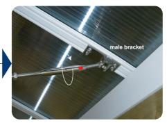
Rotate the tensioner onto the threaded stud of the male bracket, this will simultaneously draw in the terminal on the end of the wire.
