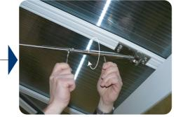
Use a tool in the hole of the tensioner to apply the final turns. A 10mm spanner on the flats of the wire terminal will stop the wire from rotating.
