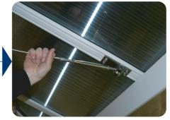
Final tension is achieved once the wire is straight and taut. Do not overtighten and allow the sides of the roof to become distorted. Tighten the locknuts against both ends of the tensioner body.
