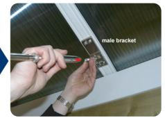
Bring the end of the wire with the tensioner across the roof to meet the **male** bracket. Offer the end of the tensioner (with the red spot) onto the threaded stud fixed to the male bracket.
